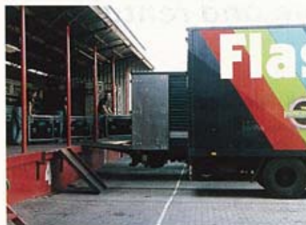
The extensive loading area.
